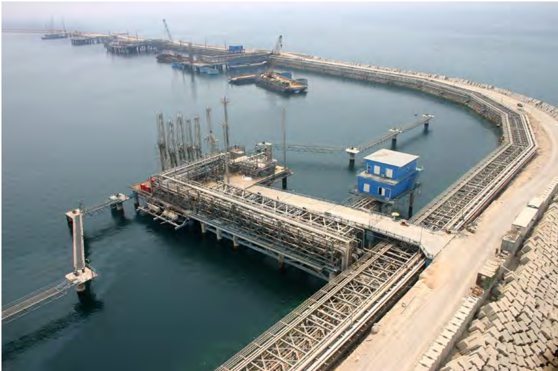
Figure 1: Pipelines passageway on the western breakwater crust at Pars Petrochemical Port
