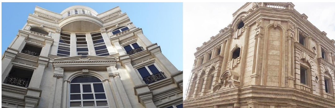
Figure 1: Applying large pieces of marble stone in façade [4]
